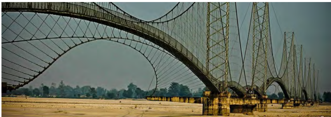
> Figure 5-33 Dodhara Chandani suspension bridge, Far Western Nepal
