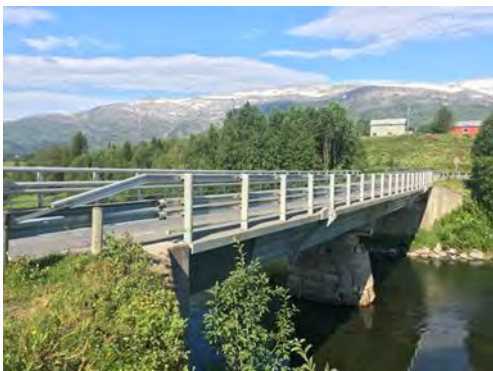
> Figure 3-2 Forsmo bridge (NTNU)
