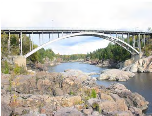
> Figure 3-1 Arvida Bridge
